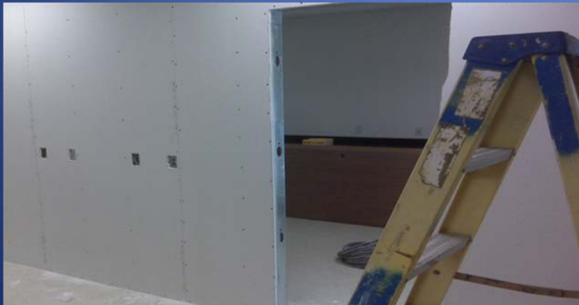
3 Dry wall installation
