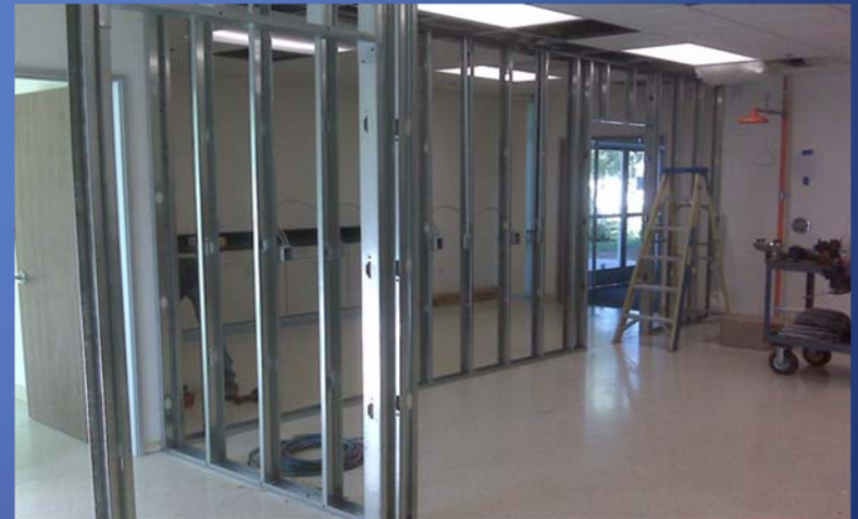
2 Framing the sample lab
