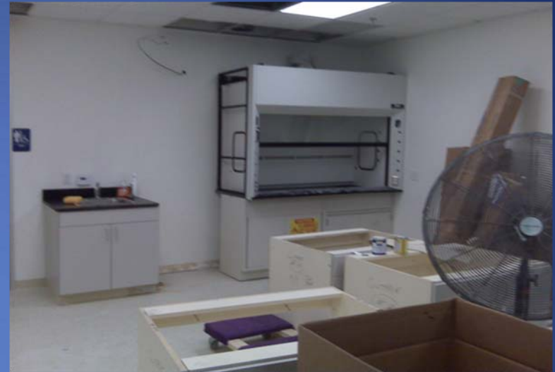
1 Hood moved for larger sink and ice maker
