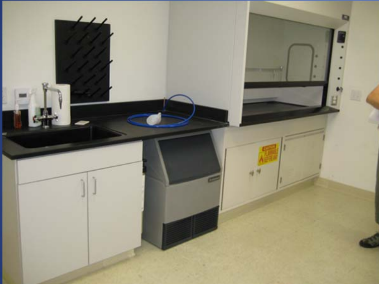
3 Ice maker installed and fittings for RO water system
